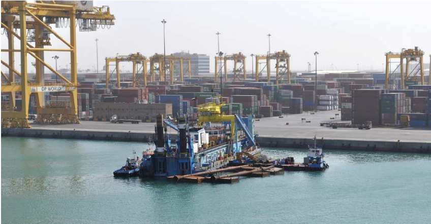
National Marine Dredging vessel dredging at Jebel Ali Port
